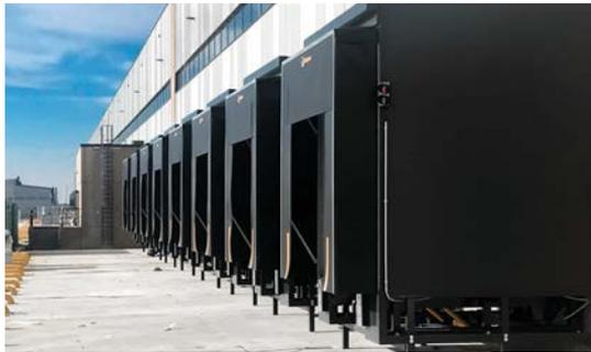
Retractable shelters installed free standing frames and dock houses.
