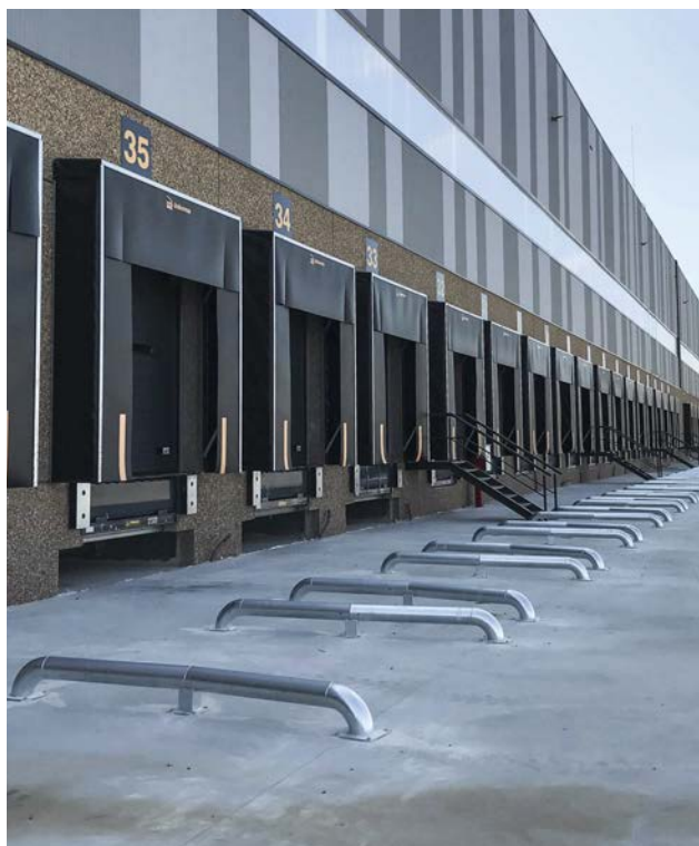
Fully galvanised reversible lorry guides.
