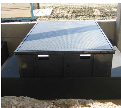
Pit for RH32 with formwork (optional)
