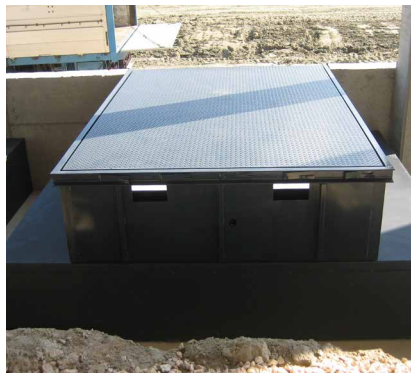
Pit for RH33 with formwork (optional)
